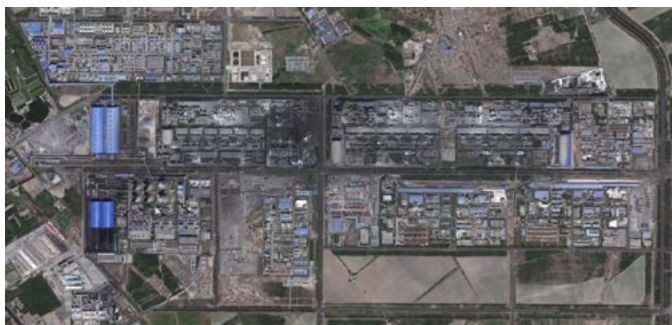
Xinjiang Tianye chemical complex in Shihezi City. 103 Coordinates: 44.35801375500167, 86.0427517885306.
