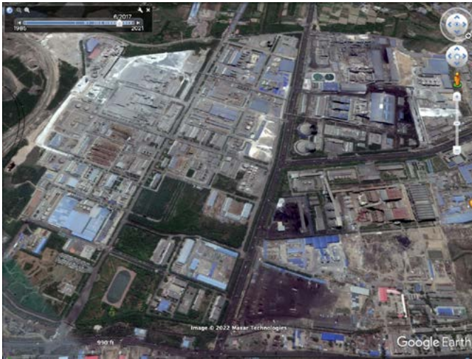
Xinjiang Huatai in the Midong District Industrial Park near Ürümqi. 47 Coordinates: 43.942935, 87.664081.
